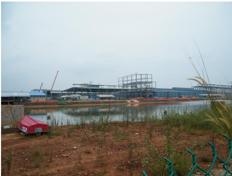
Fig. 2.4: Lynas plant seen from the west boundary with extension under construction
