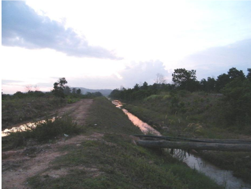
Fig. 3.10: Further path of wastewater towards Sungai Balok, approx. 3 km long
