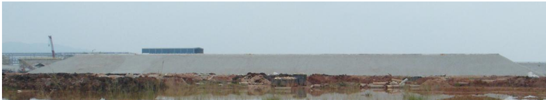
Fig. 4.3: Storage facility, phase I (photo taken October 2012)
